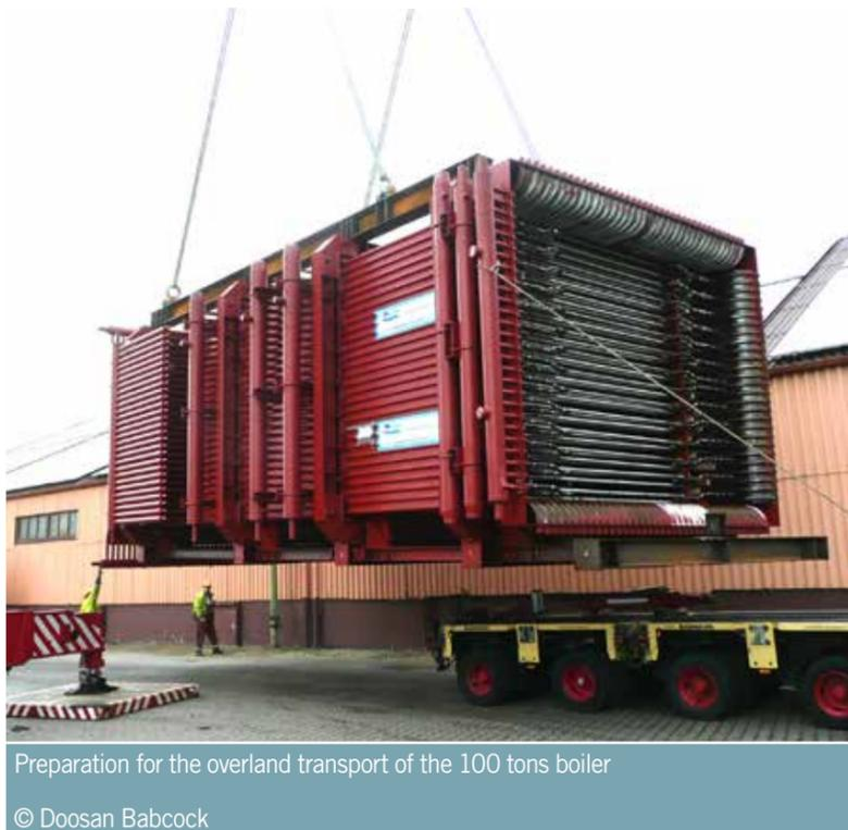
Preparation for the overland transport of the 100 tons boiler
